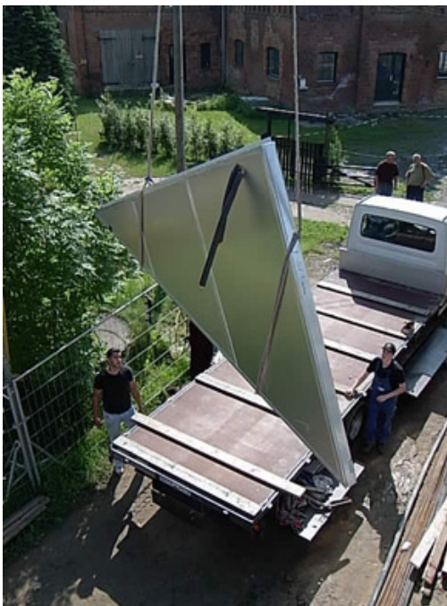
on building site – setting up solar thermal collectors
