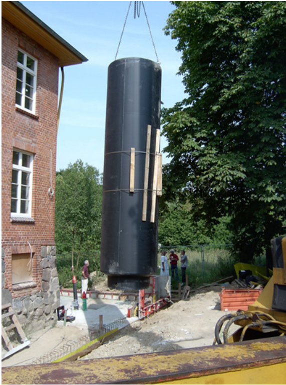
on building site – lifting storage tank on it place, finished tank in house
