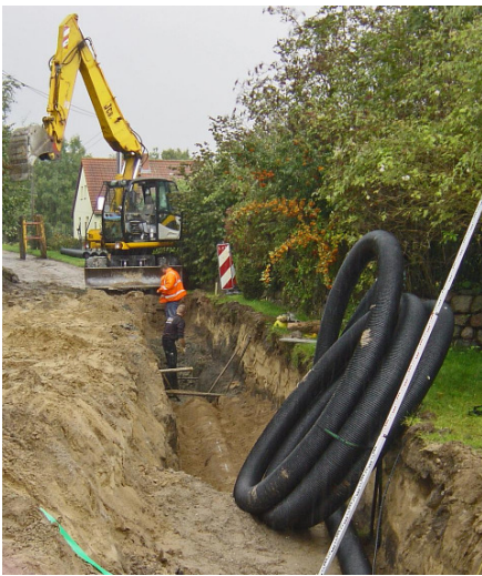
Figure 2 Installation of the heating grid
