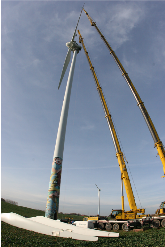
on building site – setting up rotor blades
