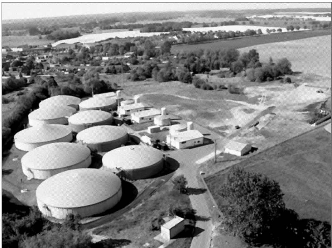
Figure: Continuous working biogas plant (Photo: Bützower Wärme GmbH)
