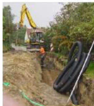
Figure 3 Installation of the heating grid
