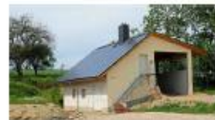
Figure 2. Wood chip heating station with storage room (2010)
