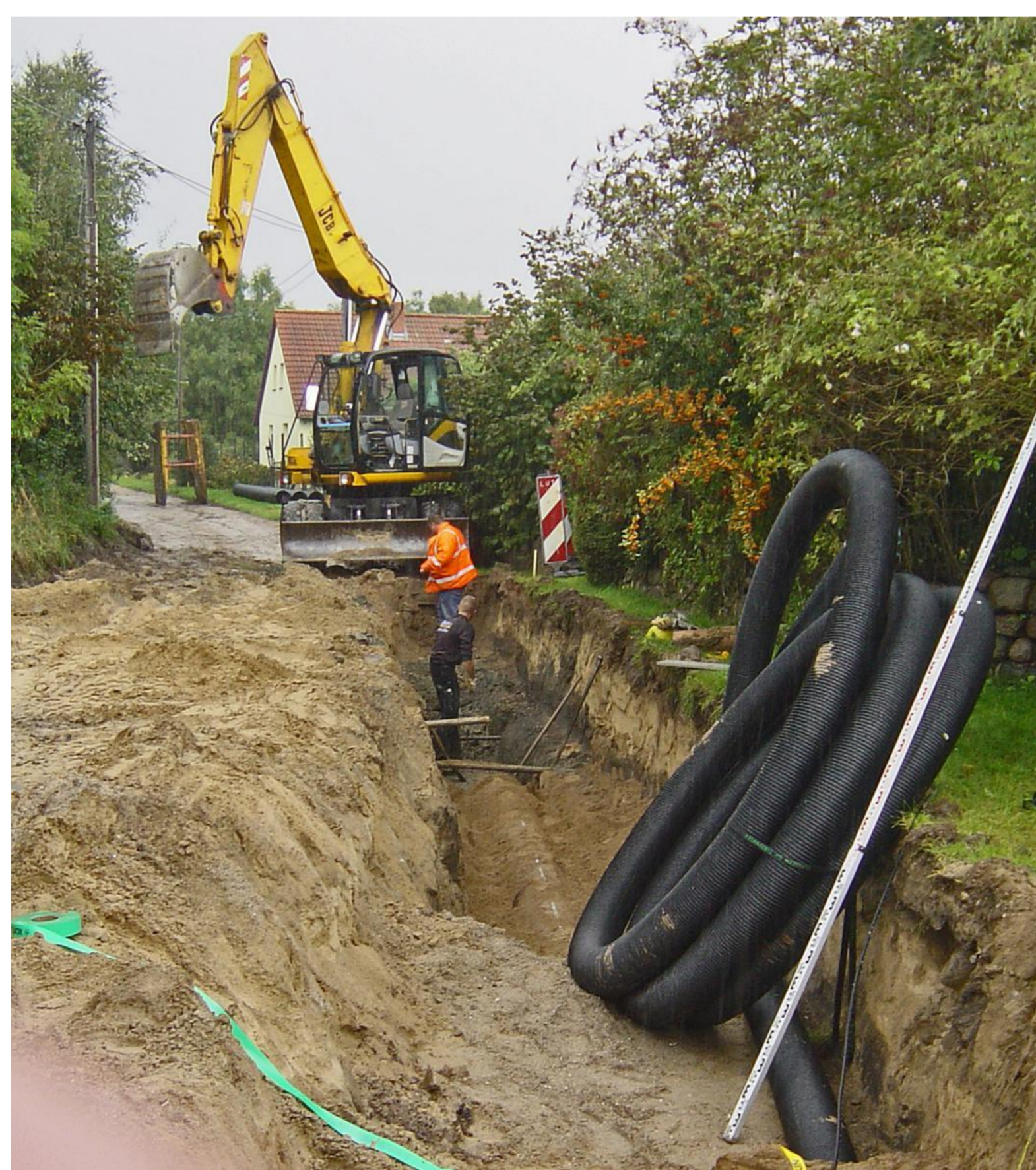
Figure 3 Installation of the heating grid
