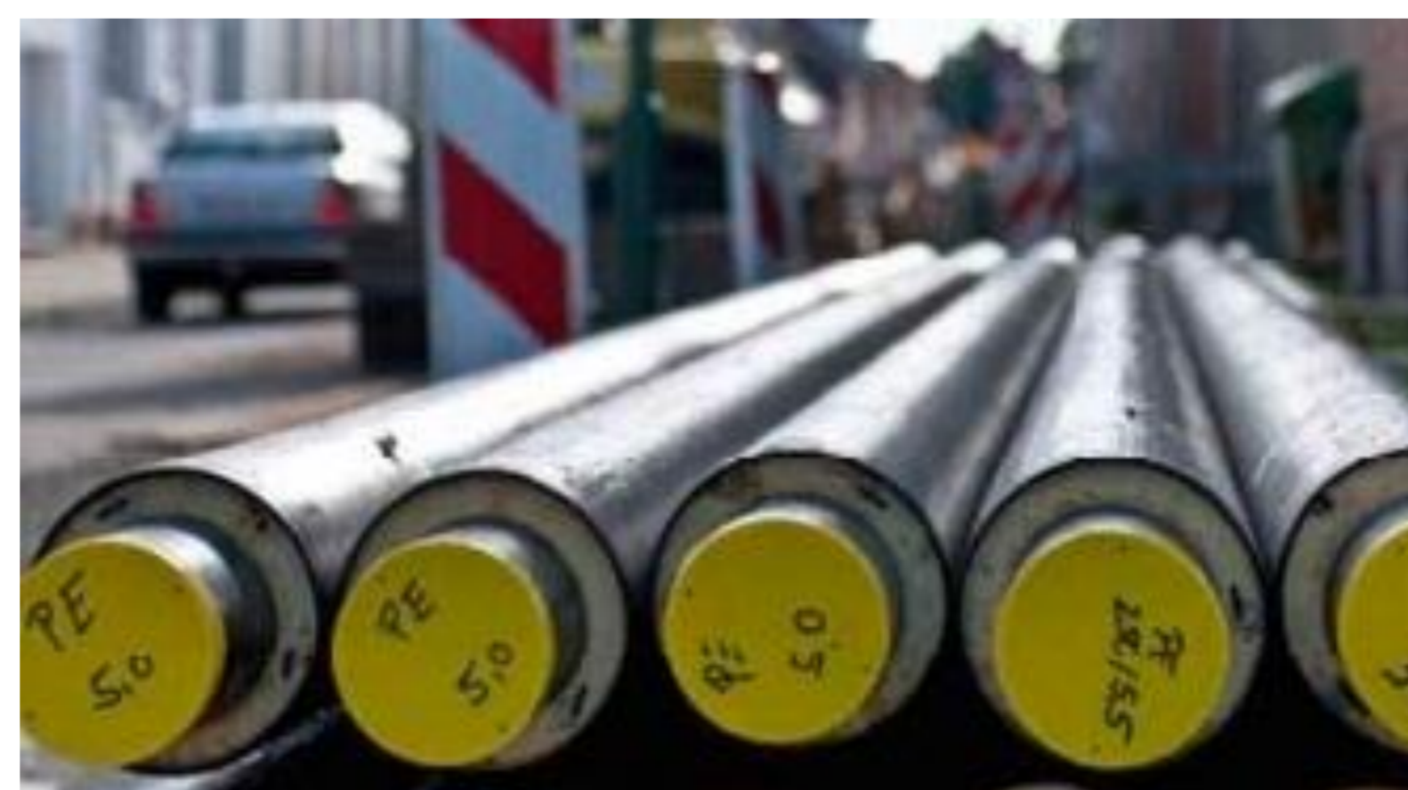
Figure 3 pipes for the new grid
