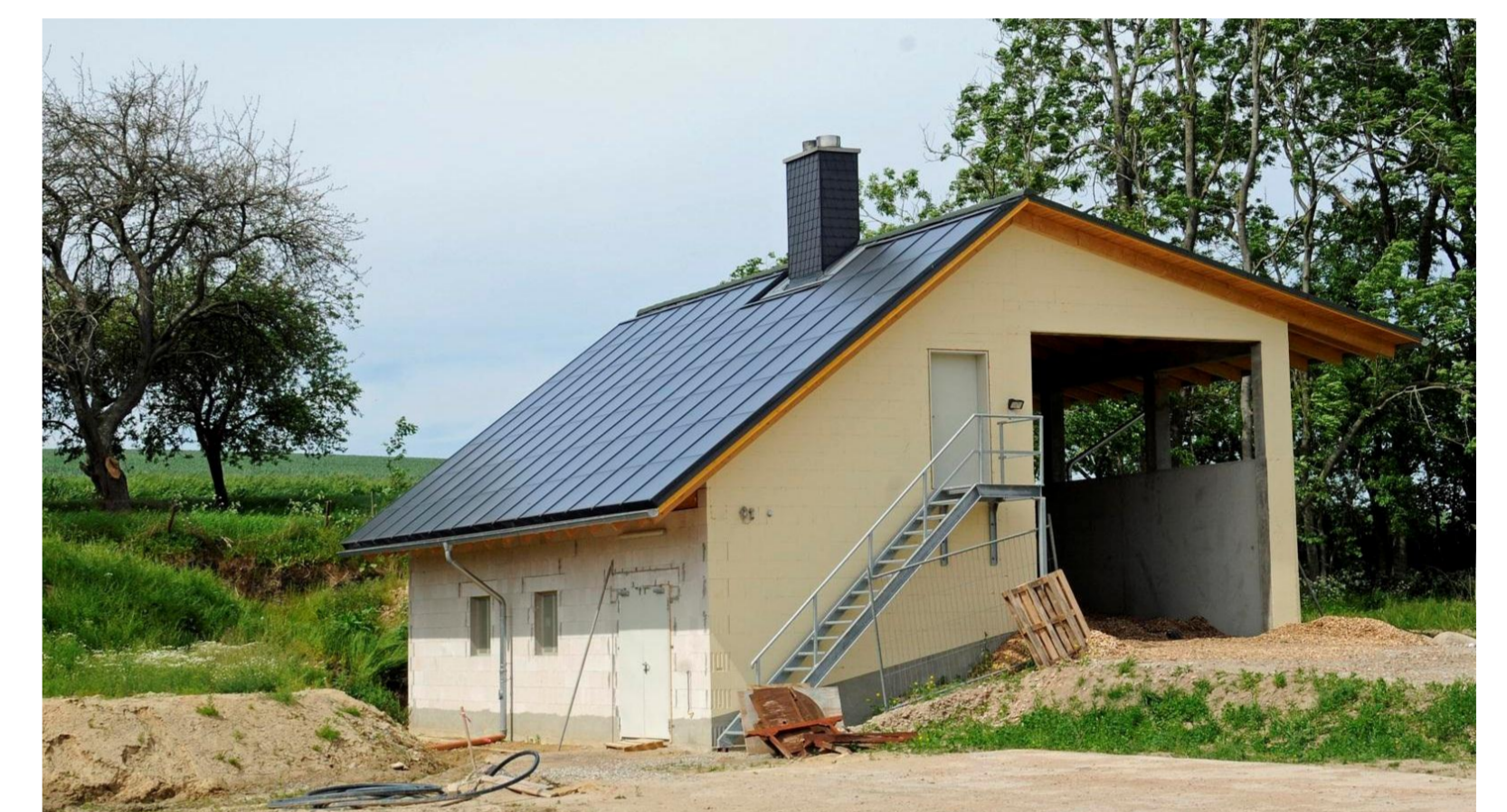
Figure 2. Wood chip heating station with storage room (2010)
