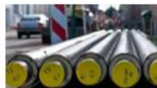
Figure 3 pipes for the new grid
