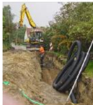
Figure 3 Installation of the heating grid
