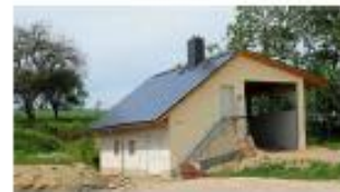
Figure 2. Wood chip heating station with storage room (2010)
